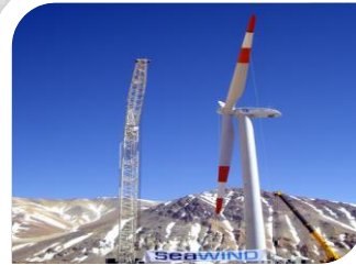
Adapted, erected & maintained the utility scale wind turbine, suitable for high altitude
